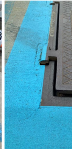
Cracked Hold Open Arm
